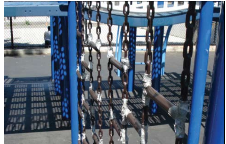
Russell Pederson Park, Brooklyn: Sloppy maintenance conditions were frequently found on playgrounds, affecting 81% of surveyed sites.
