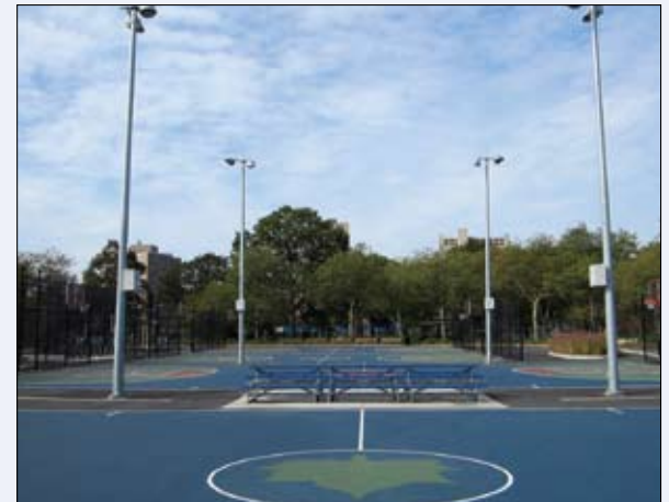
New basketball courts with lighting.
