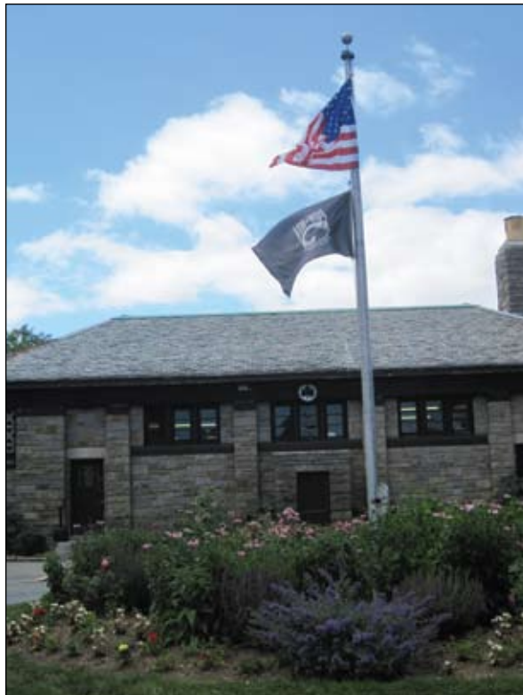
Alley Park Recreation Center
