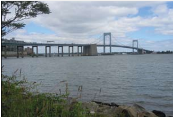
Little Bay Park provides scenic views of Little Bay and Throgs Neck Bridge.
