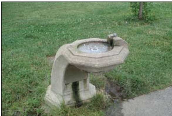
Standing water and overflow have caused algae to form in the basin and along the base of this fountain.
