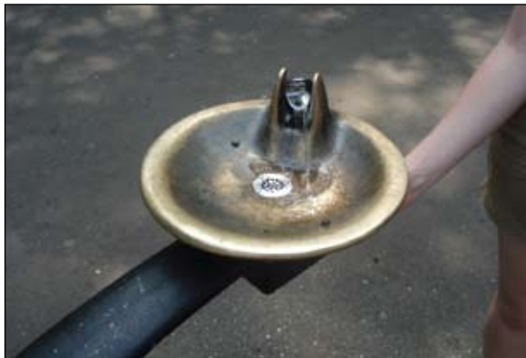
Drinking fountains were in excellent condition.
