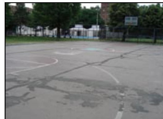
Corporal Thompson Park, Staten Island, 2006. This basketball court is missing sections, providing an unsafe play area.
